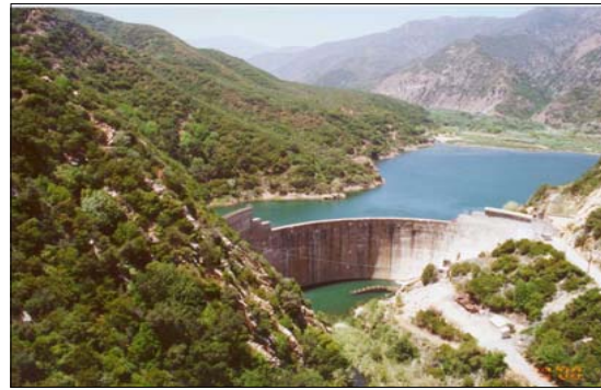
Matilija Dam and Reservoir
